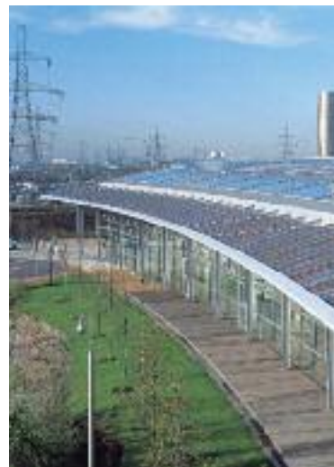
PV system integrated on a roof.
