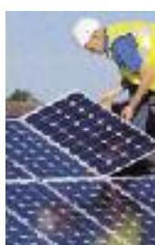
Worker installing PV module, Wesco court, Woking, UK.
