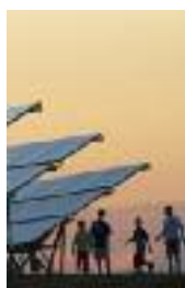
Erlasee Solar Park, one of the largest tracking PV solar power station in the world.
