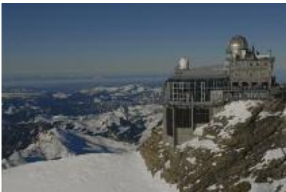
Off-grid industrial application.
