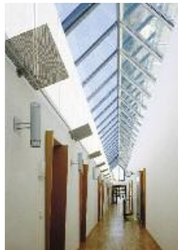
Glass roof, a-si amorphous silicon thin film integrated in glass.
