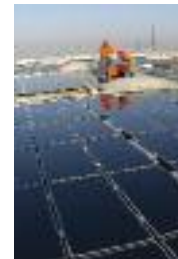
Installing thin film modules.
